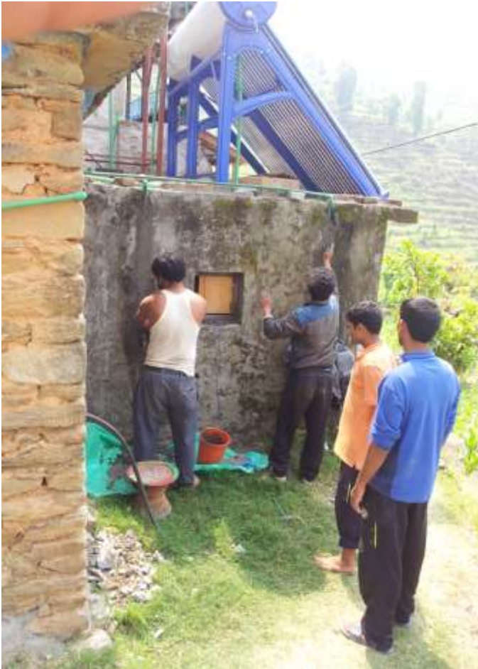
Picture 7: Covering the pipes with cement
