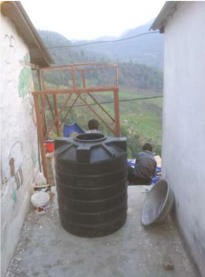
Picture 3: Tank stand was installed
