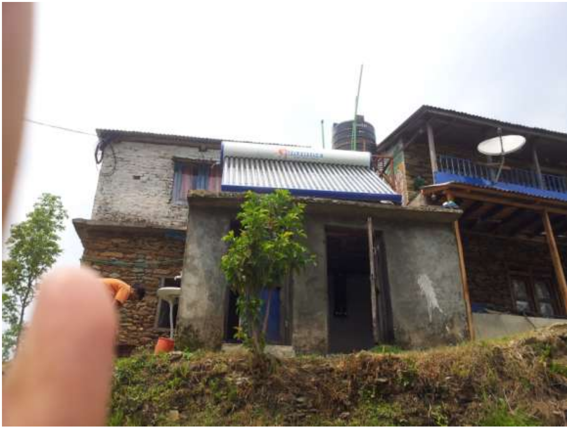
Picture 10: After the installation was complete
