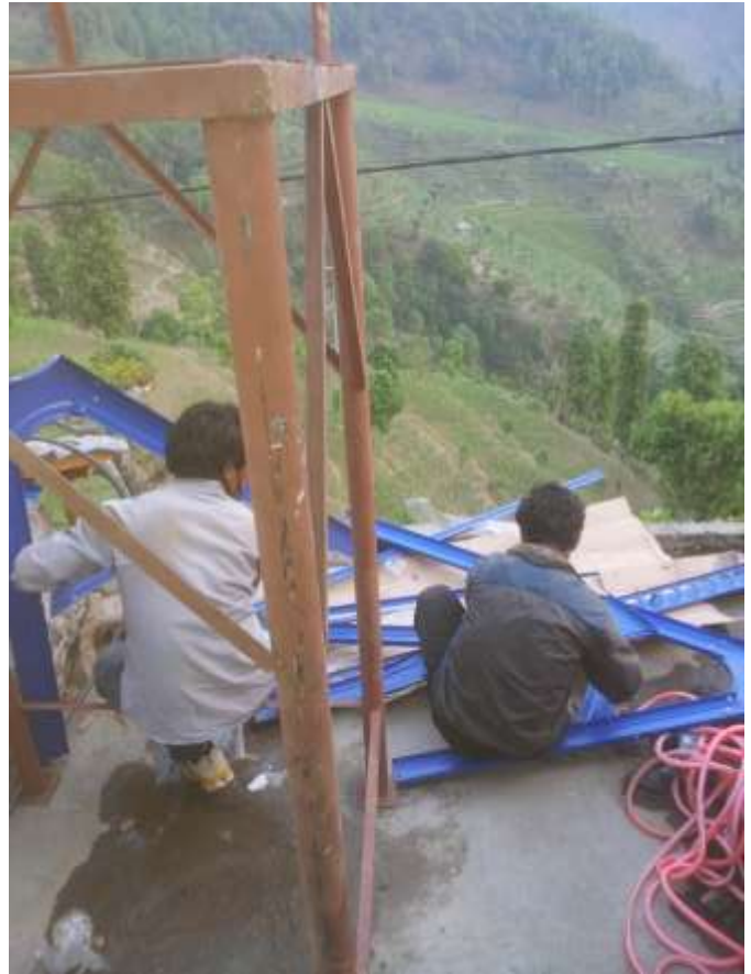
Picture 2: Frames were set up
