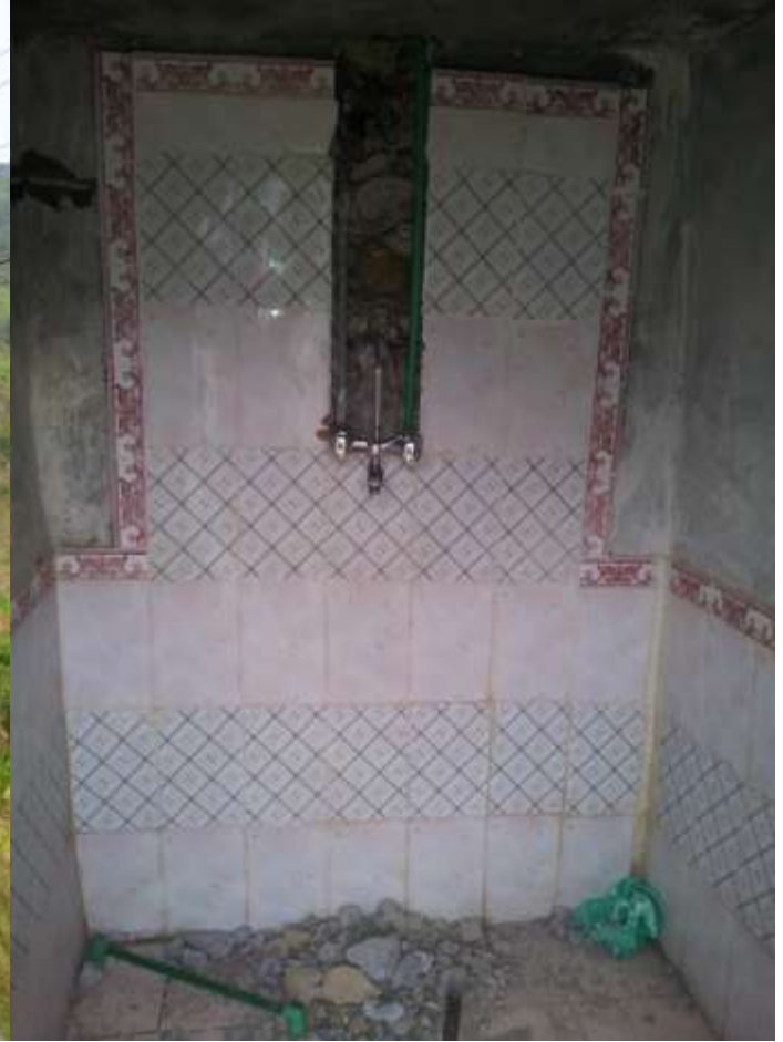
Picture 5 Tiles were broken off to install the mixture
