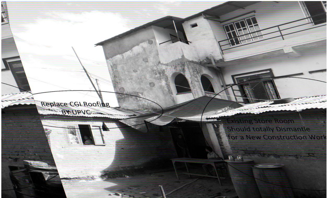
Existing Structures in place
